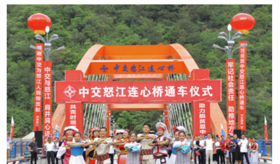
2020 年 8 月 12 日，中交怒江连心桥正式通车 On August 12, 2020, CCCC Nujiang Heart Connection Bridge is formally opened to traffic
