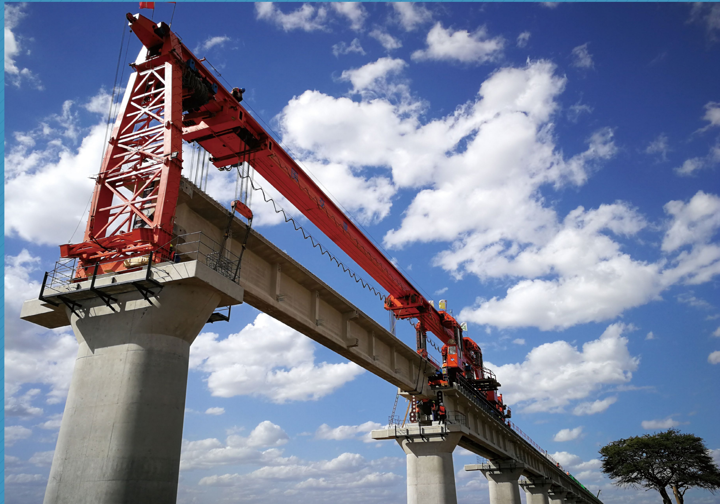
内马铁路铺架 Track laying and girder erecting
