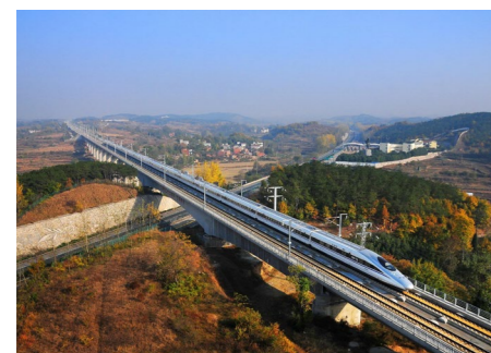
京沪高速铁路 Beijing-Shanghai High-speed Railway
