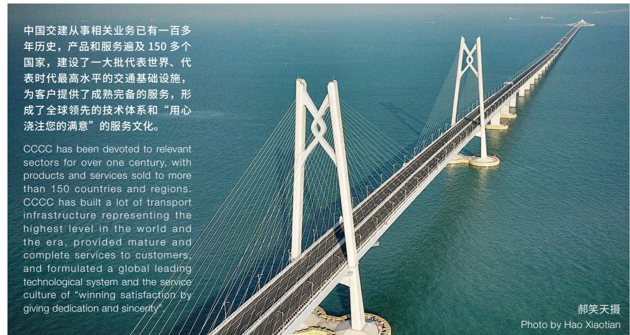
港珠澳大桥青州航道桥 The Qingzhou Channel bridge of Hong Kong-Zhuhai-Macao bridge
